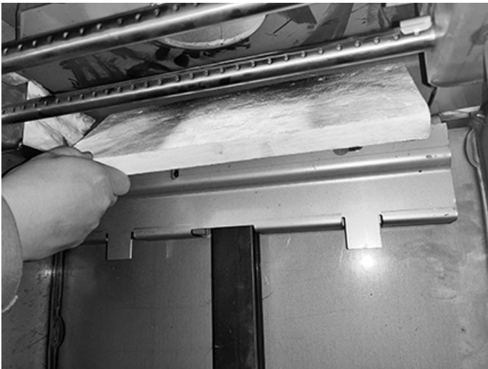
Figure 3: Baffle board removal.
